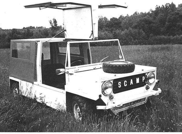
Having reached a production total of around 700, the first-generation Mini-Scamp was replaced by a Mk. 2 model in 1978. As ever, running gear was from the good old Mini, the main changes being in the bodywork department and with a stronger multi-tubular chassis. The Mini-Scamp Mk. 2 is still available at the time of writing, although the gullwing doors have been replaced by doors hinged in the normal fashion.
